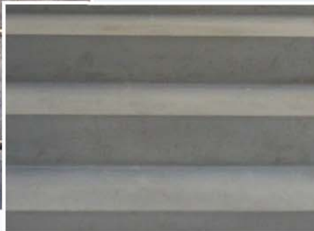
Precast Concrete Stair
